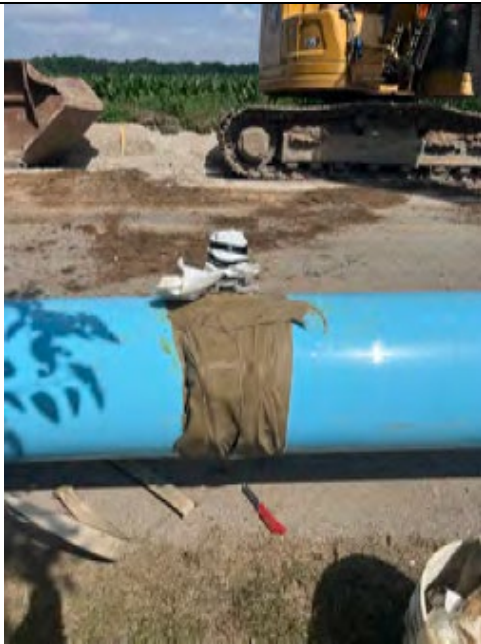
ARV saddle with Denso tape ready for installation
