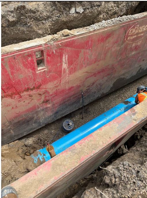
Open cut watermain installation in progress
