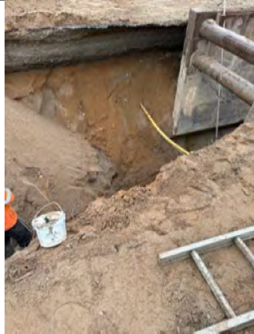
Preparation to install watermain below a gas line
