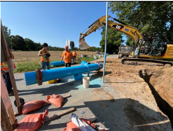
Open cut watermain installation along Falconbridge Road
