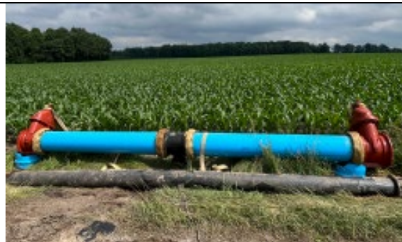
Gate valves and Tee connection prepared for installation
