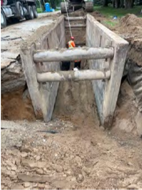
Trench box for open cut watermain installation on Falconbridge Road
