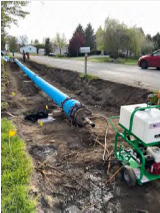
HDD pipe being pressure tested prior to installation
