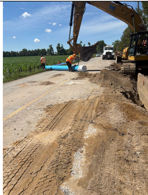
Watermain pipe prepared for installation
