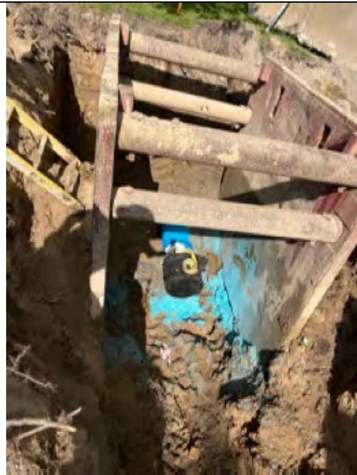
Trenchless pipe installed ready for connection
