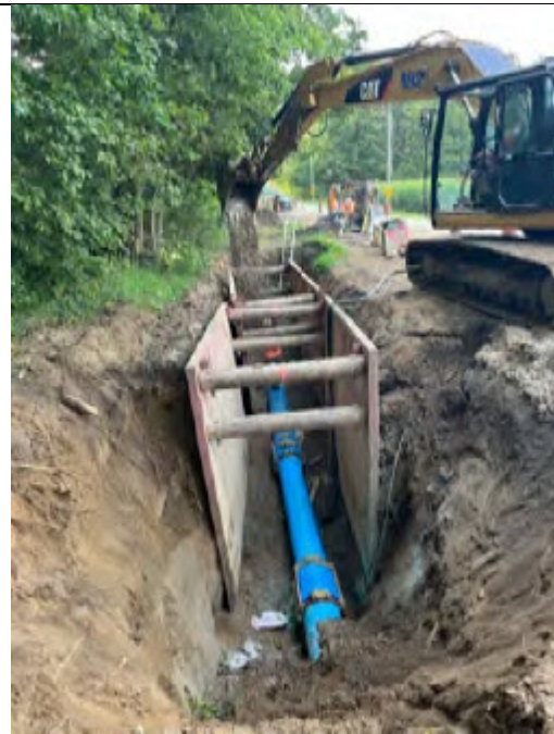
Trenchless pipe installed ready for connection
