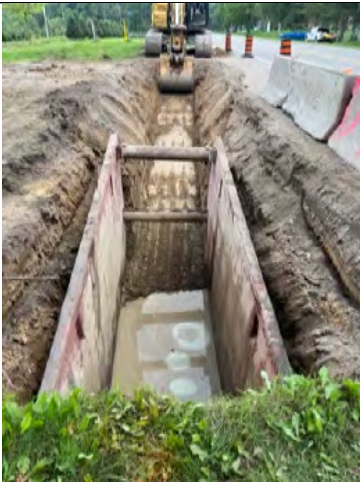
Receiving pit and sloped trench on Longwoods Road
